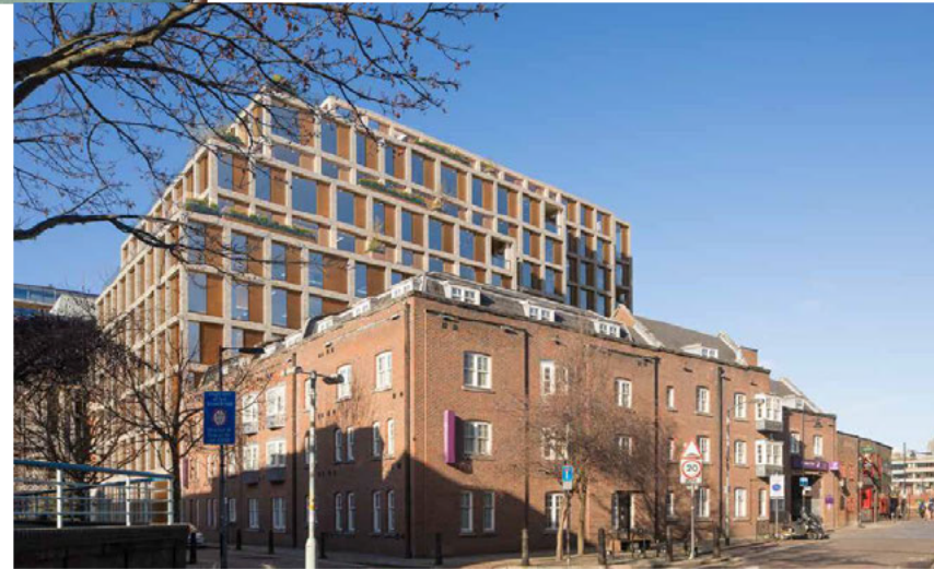
View from Park Street, corner with Bank End looking at the Premier Inn
