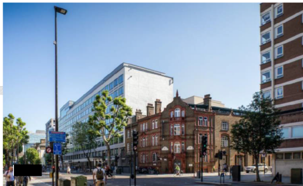
View from Blackfriars Road
